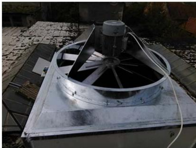
Fig. 5. Fan of presented cooling tower
